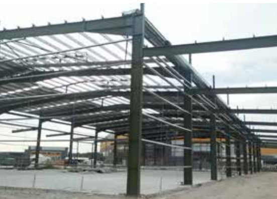
Iskandar Malaysia Studios Sdn. Bhd. Steel Structural Works
