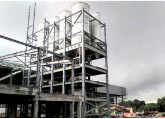
Quic-Seal Construction Chemicals Sdn. Bhd. Steel Structural Works
