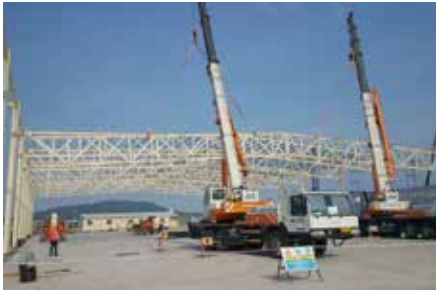
55 Tons & 25 Tons Mobile Cranes
