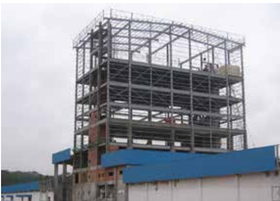
Super Food Specialists (M) Sdn. Bhd. Steel Structural Works
