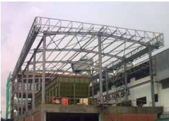
Southern Lion Sdn. Bhd. Steel Structural Works
