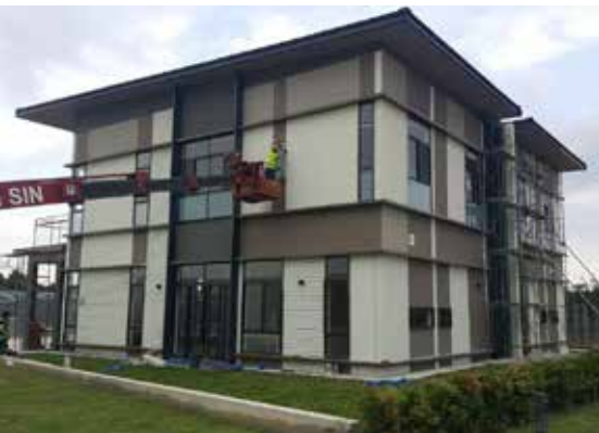
Daiwa Sunway Development Sdn. Bhd. Steel Structural Works
