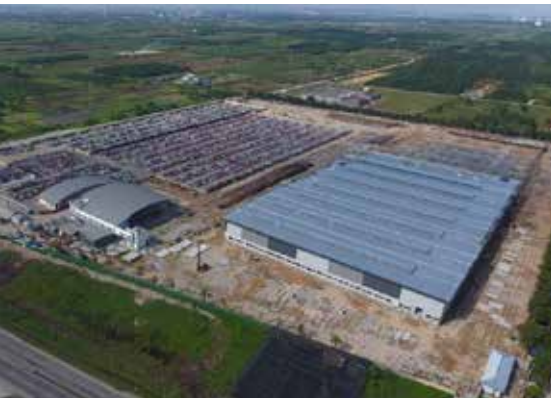
Axis Reit Steel Structural Works
